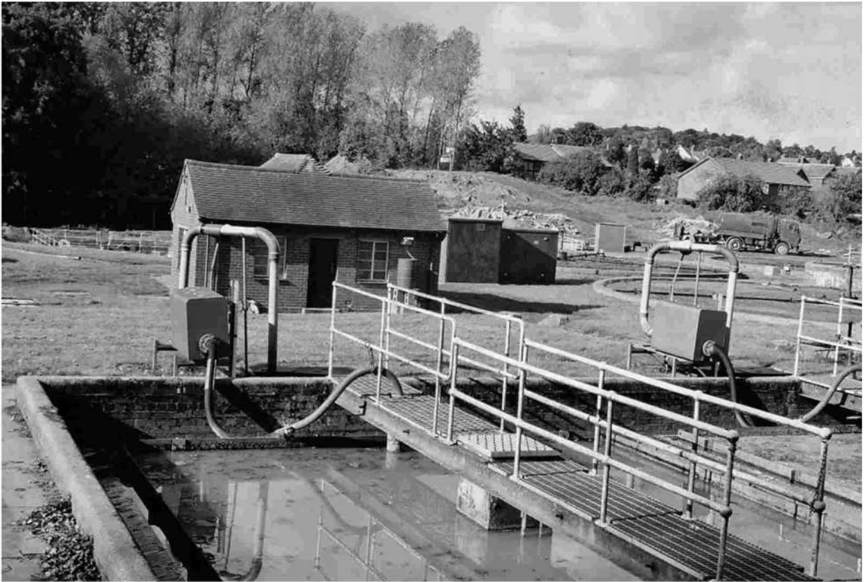
Pumping Station and Sedimentation Beds
