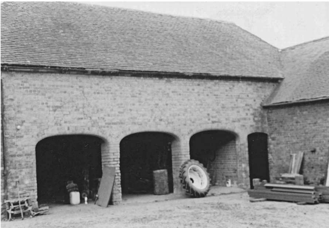
Cart shed at Brakemill Farm with a granary above for storing grain after it had been threshed
